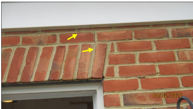
cracking mortar
