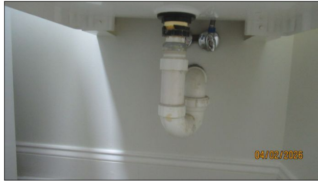
drain leak
