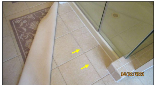
deteriorated grout
