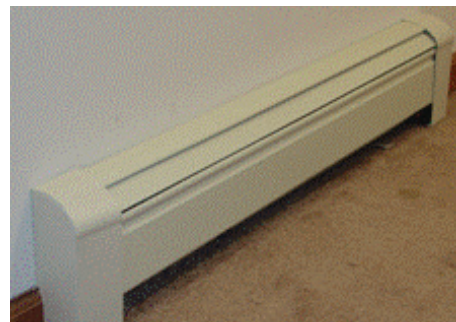
Hot Water Baseboard Register
