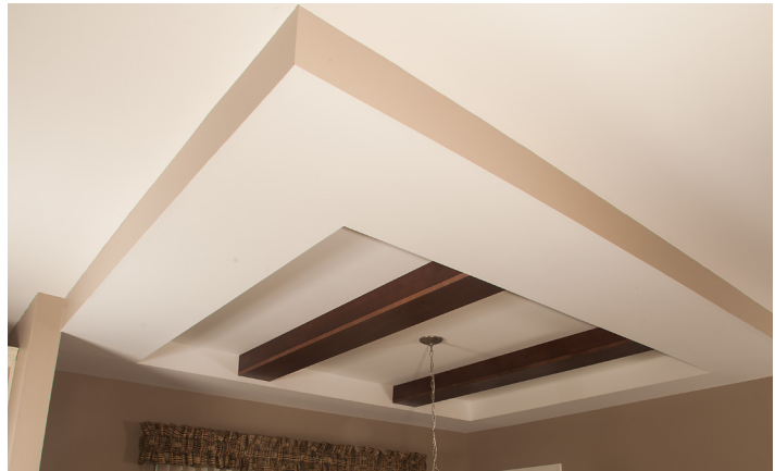
Tray Ceiling with Wood Beams
