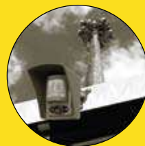
Protect Cell Towers
