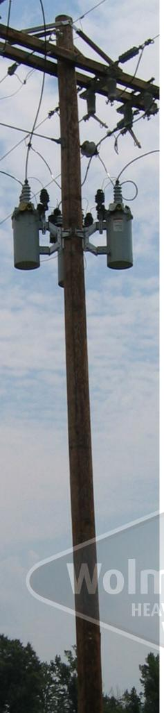
Following treatment with Wolmanac® CCA, utility poles produced by Desoto Treated Materials receive an extra treatment penetrating the outer layer with ET® Brown oil emulsion. This emulsion serves as a lubricant, making the pole easier to climb and service, without affecting the preservative properties of the CCA treatment.
