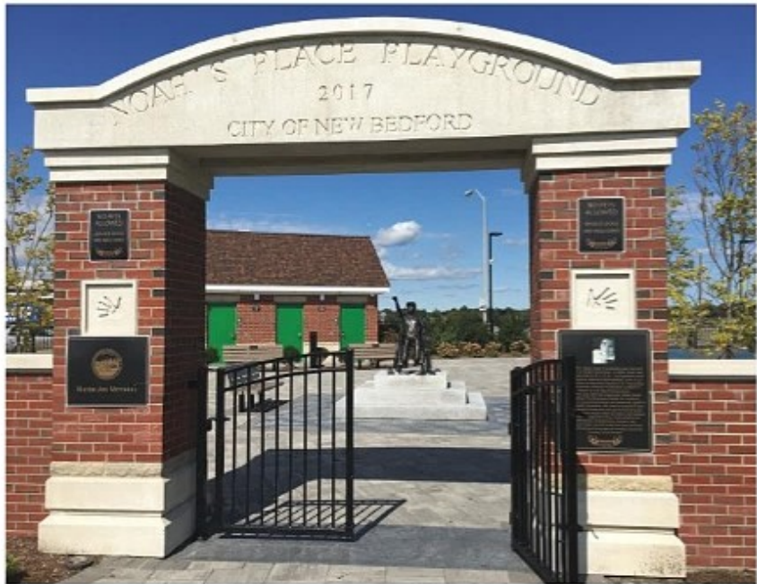
Located in New Bedford, Massachusetts, Noah's Place Playground is an interactive playground for children with disabilities. Breault Roofing, Inc. provided the crane service to install the massive stone sign at the entrance to the playground.
