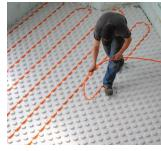
NUDURA has brought innovation to the market with our line of Insulated Concrete Forms, that innovation continues with HydroFoam™. Installation is fast and easy compared to traditional foam insulation which requires multiple steps to run radiant heat piping. The 4' × 4' (1.2 m × 1.2 m) boards, available in two thickness, are easily installed with an overlapping interlock on all four sides, ensuring the boards are locked in
