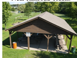
Near Railroad Tracks
