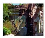
Our remedy was to first remove the efflorescence with ACON Efflorescence Remover, and then we applied ACON Deep Seal to the wall. The result is that the park has enjoyed several years of efflorescence free walls, with no damage to the mural.
