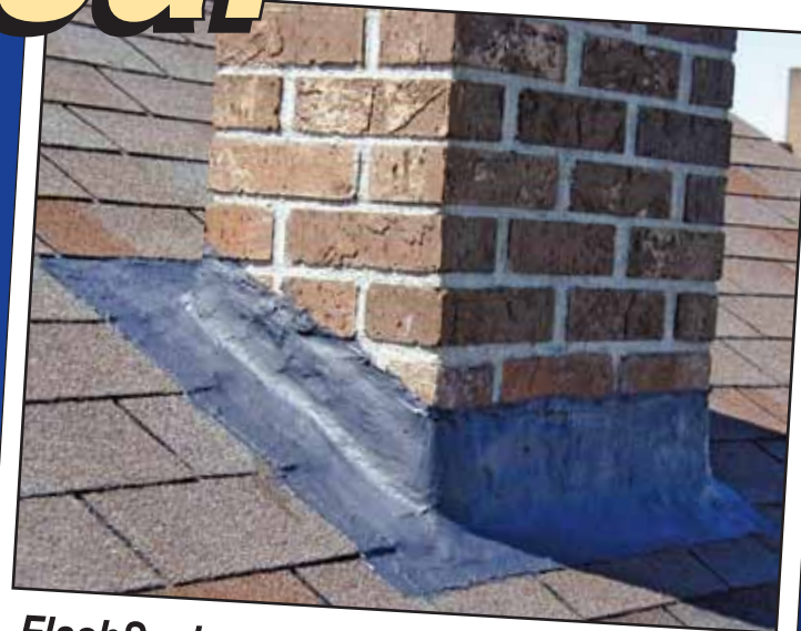
FlashSeal repairs faulty flashings around chimneys, stacks, and vents
