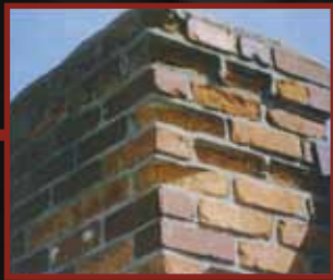
Spalled Bricks
