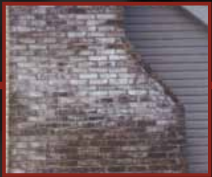
Efflorescence
