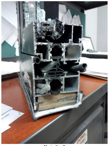
**Photo No. 3**Section view of sill detail
