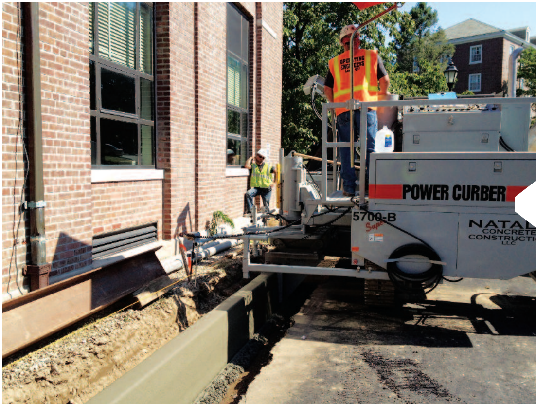
Nick Natale's rebuilt 5700-Super-B is perfect for pouring in tight spaces.
