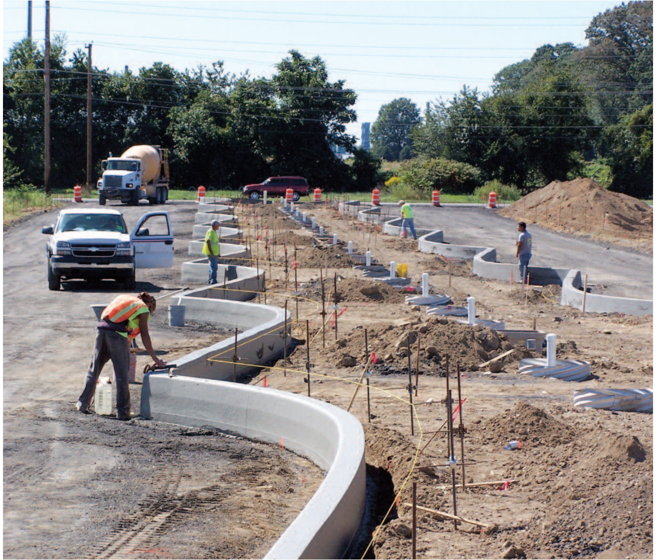
Multiple radii poured with 5700-C on bus terminal job site in Dover, DE.
