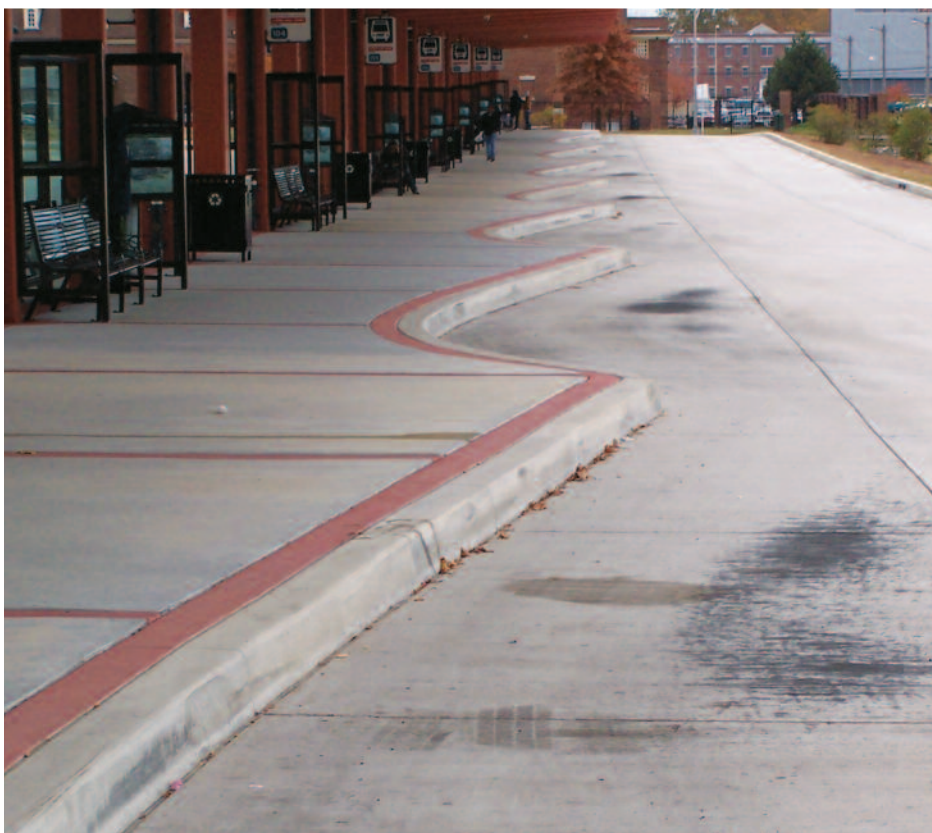
Finished project, and a job well done.
