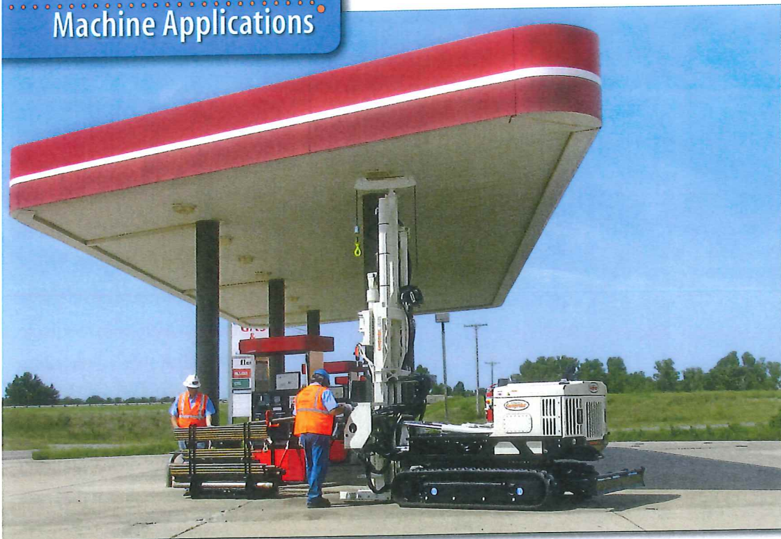
Underground Storage Tank Investigations At this site, the 7822DT is used to collect soil and groundwater samples to determine the extent of contamination from a leaking underground fuel line.
