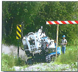
A 7822DT onsite makes small work of rugged terrain and barricades.
