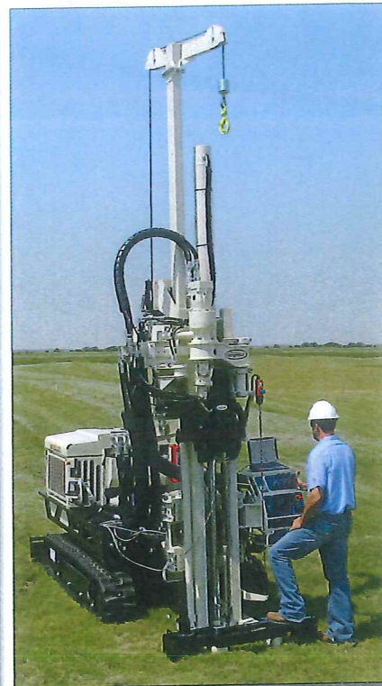
Cone Penetration Testing CPT testing is a common application for 78 Series machines. The augerhead torque allows insertion of ample-sized anchors to stabilize the machine. Up to 9 tons of push is typical for this platform. Once the CPT cone has been pushed and recovered, the operator is able to change functions and perform confirmatory soil sampling with the same machine.
