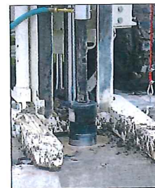
Concrete Coring A 5-in. concrete core opens up the subsurface for sampling or monitoring well installation.
