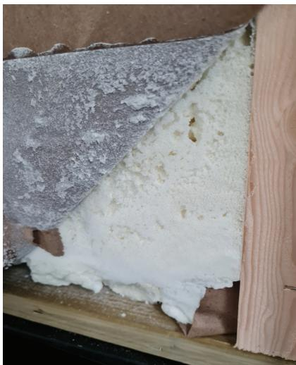
Insulated wrap with full foam insulation
