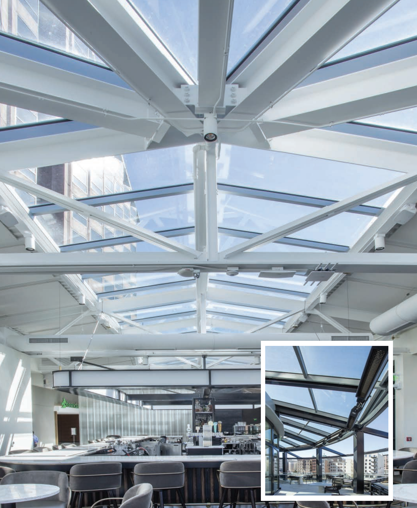
Associated Bank, River Center - Milwaukee, WI Architect: Rinka Chung Architecture
