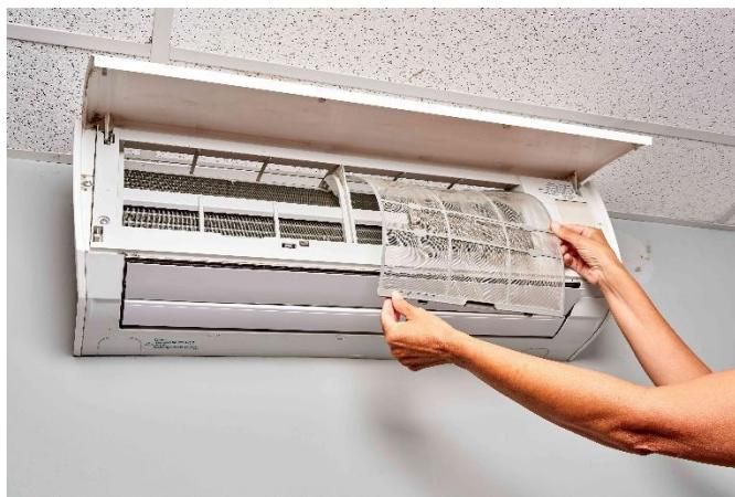
Wash them in a sink with warm water but **DO NOT USE ANY SOAP OR DETERGENTS**. Be sure to let the filters dry completely before reinstalling. If you put wet filter in, they will drip and could cause an airflow restriction and cause the unit to ice up in cooling mode or go into a fault.
