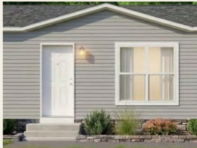
Dormer Gable over Door
