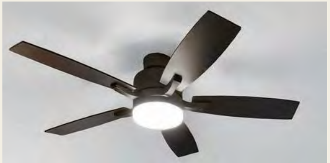
Black 5 Blade Ceiling Fan Installed
