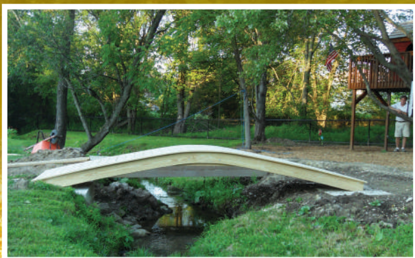
16' Wood Bridge Without Railing
